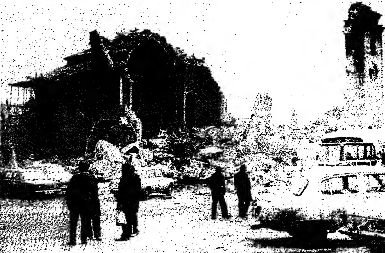
Some stunned residents of Leninakan viewing the shattered remains of the centuries-old cathedral in the centre of Armenia's second largest city yesterday.
